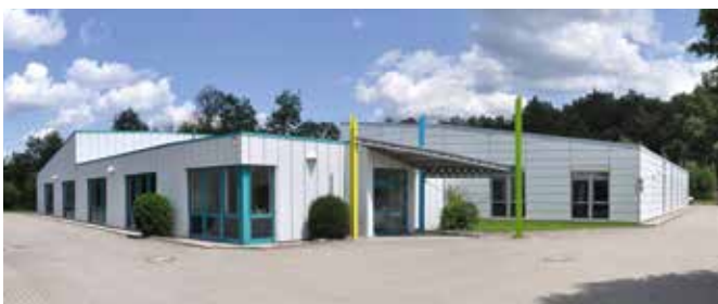
Headquarters of PHYSIOMED ELEKTROMEDIZIN AG in Laipersdorf near Schnaittach
